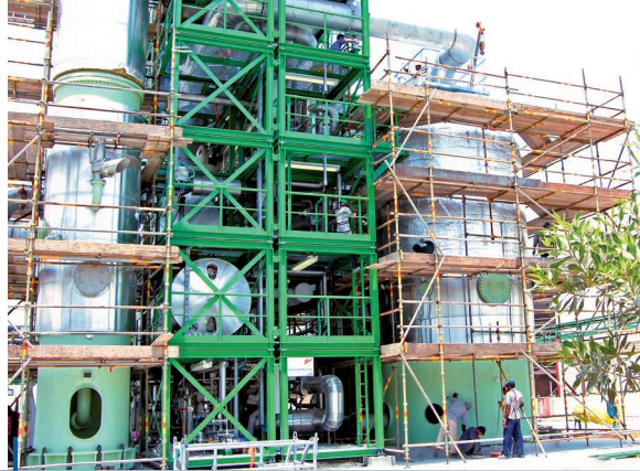
Stand-alone unit operated by Green Power WLL, Kingdom of Bahrain, comprising a pre-assembled skid, a rectification column with a reboiler and molecular sieve vessels
