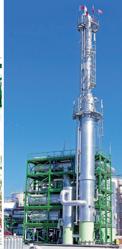
Stand-alone unit operated by Green Power WLL, Kingdom of Bahrain, comprising a pre-assembled skid, a rectification column with a reboiler and molecular sieve vessels
